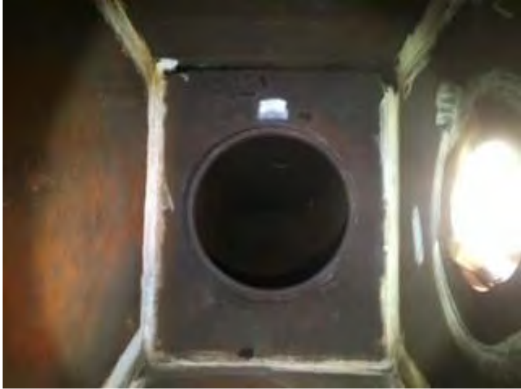
PHOTOGRAPH NO. 9 – GENERAL VIEW OF RH340B BOOM
